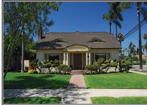
631 N. Zeyn St., Anaheim Colony This immaculate home is nearly 2,200 square feet on 6,577 square foot lot located on a pride of ownership street in the Anaheim Colony Historic District! This colonial revival beauty has graced a page of a professional calendar! $679,900
